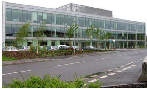
Example of a typical large scale industrial use
